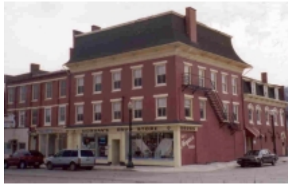
Benner Building originally constructed in 1810 was remodeled in 1876. At this time the flat roof was elevated to an empire or mansard style.
